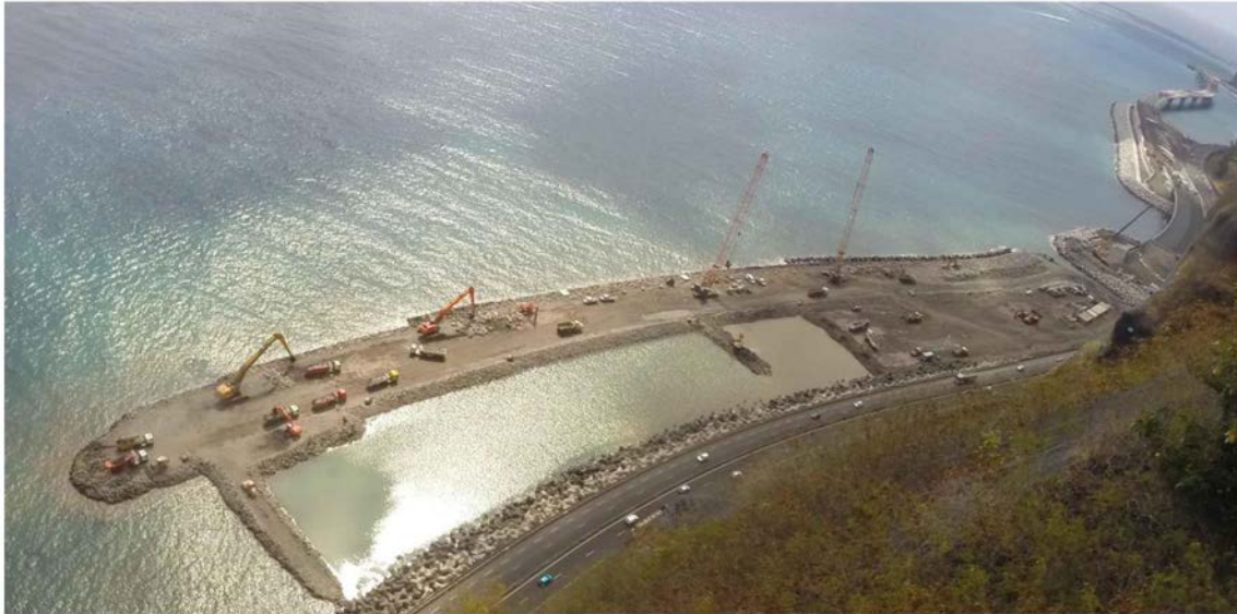
Figure 4—Dike D3 under construction
