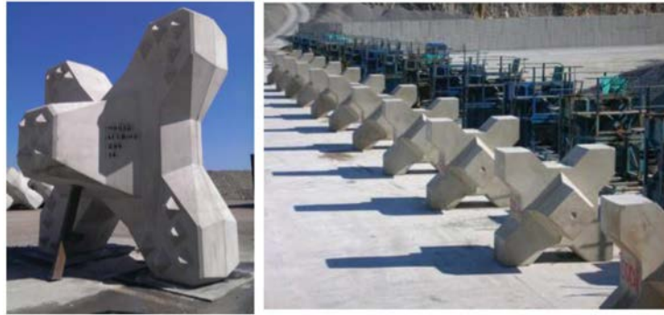
Figure 1—Typical concrete armour units used on the project NRL
